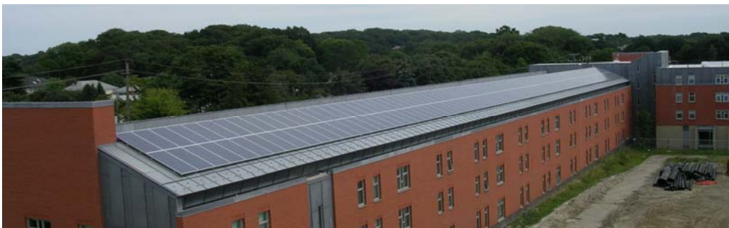
ATLANTIC HALL PHOTOVOLTAIC ARRAY SALEM STATE UNIVERSITY
