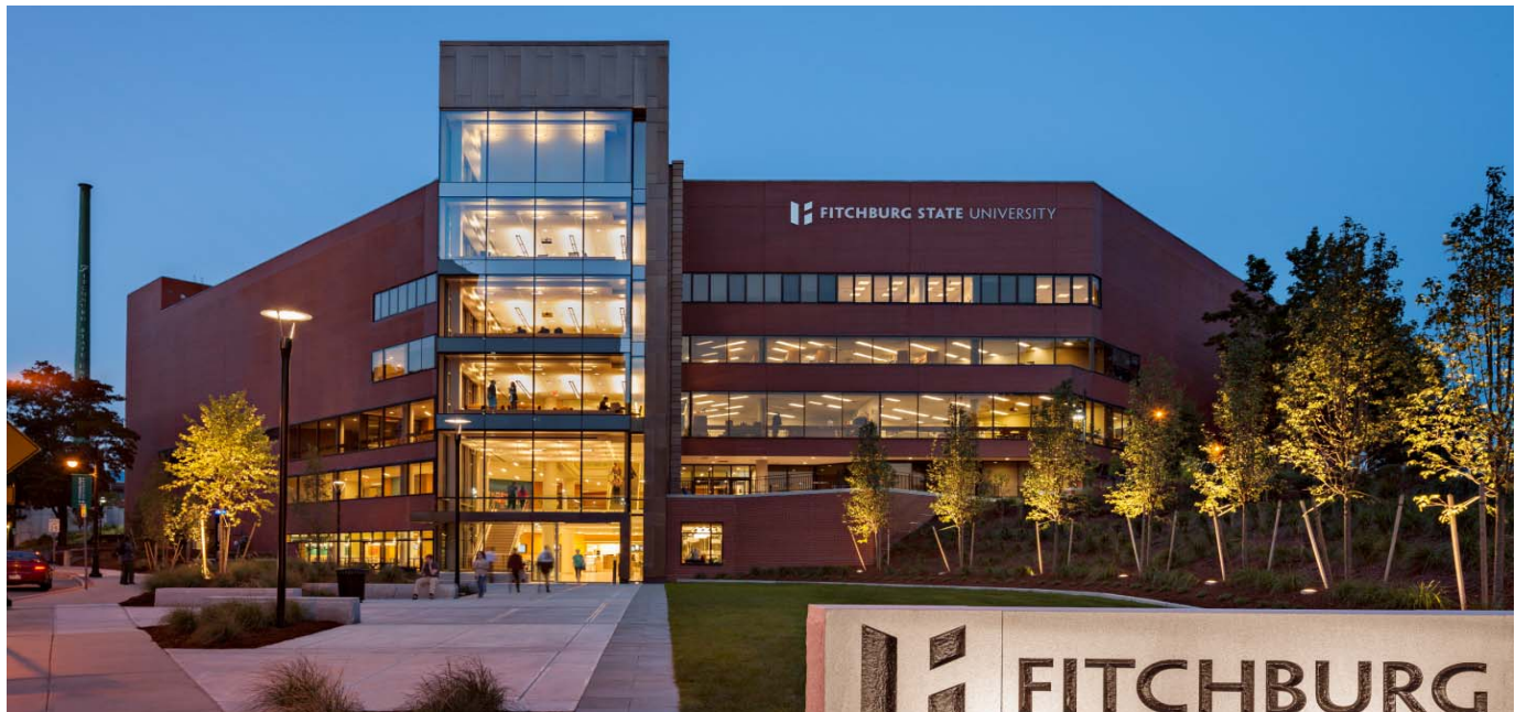
HAMMOND CAMPUS CENTER AND LIBRARY FITCHBURG STATE UNIVERSITY
