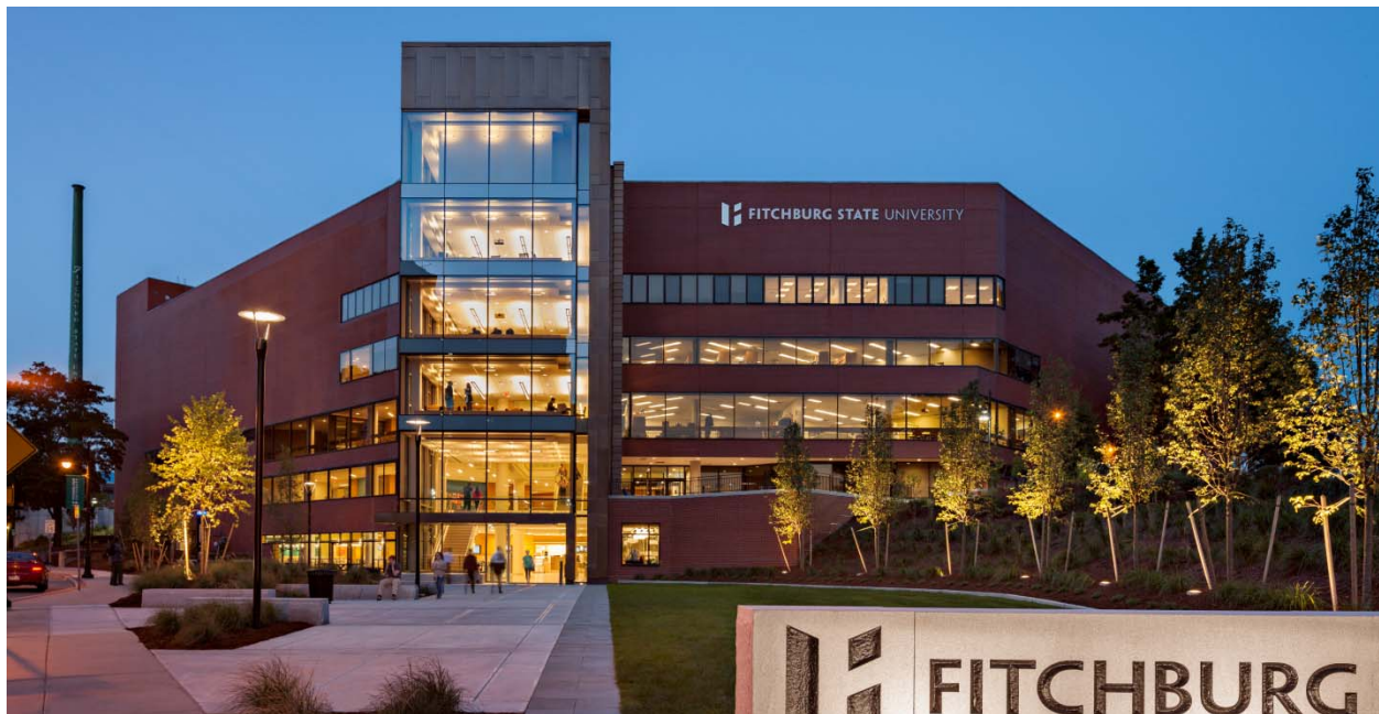
HAMMOND CAMPUS CENTER AND LIBRARY FITCHBURG STATE UNIVERSITY
