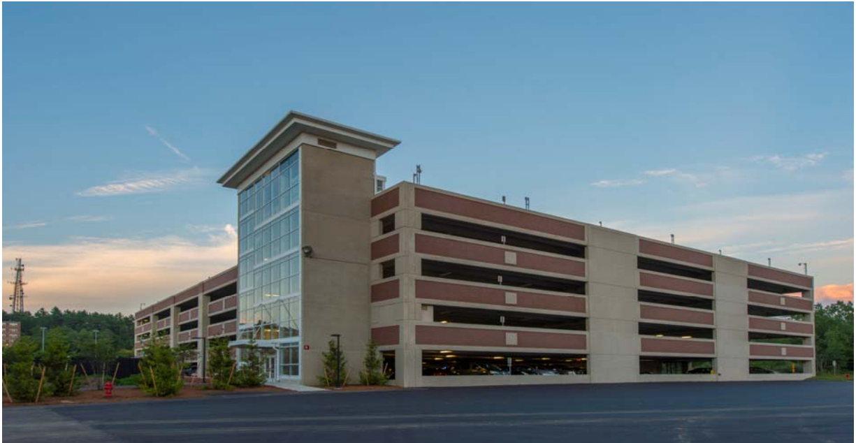
PARKING STRUCTURE BRIDGEWATER STATE UNIVERSITY
